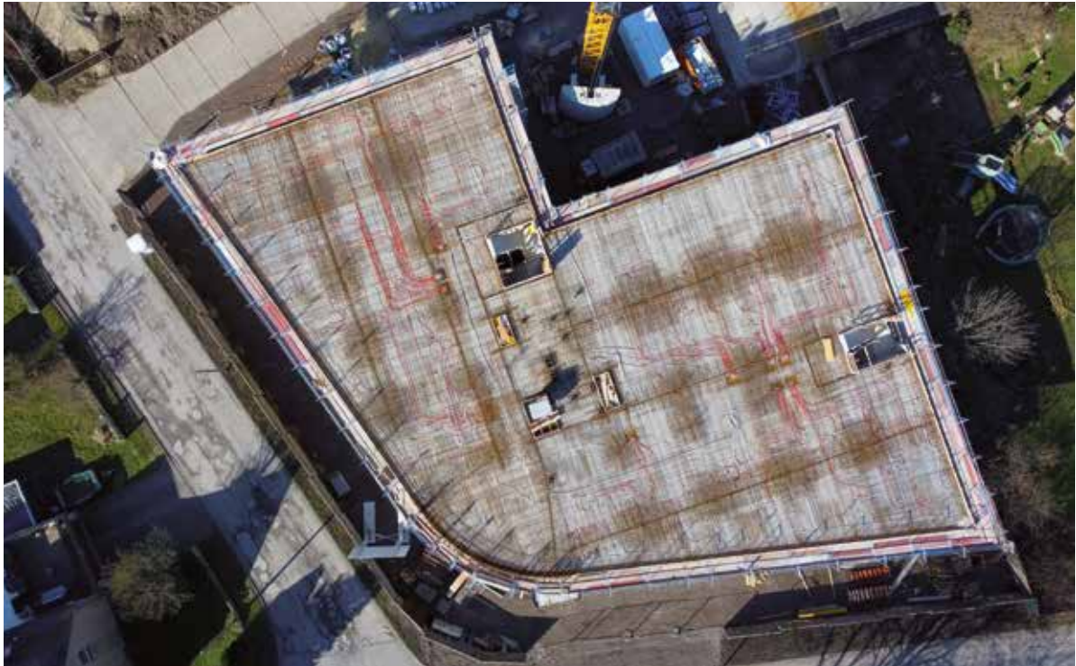
© Heitfeld Baugesellschaft mbH
